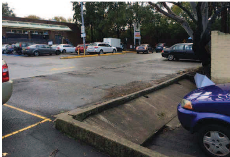
Photograph 2 – Low height retaining structures
