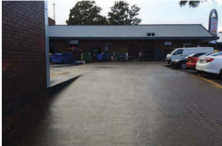
Photograph 3 – Ramp to the loading dock area
